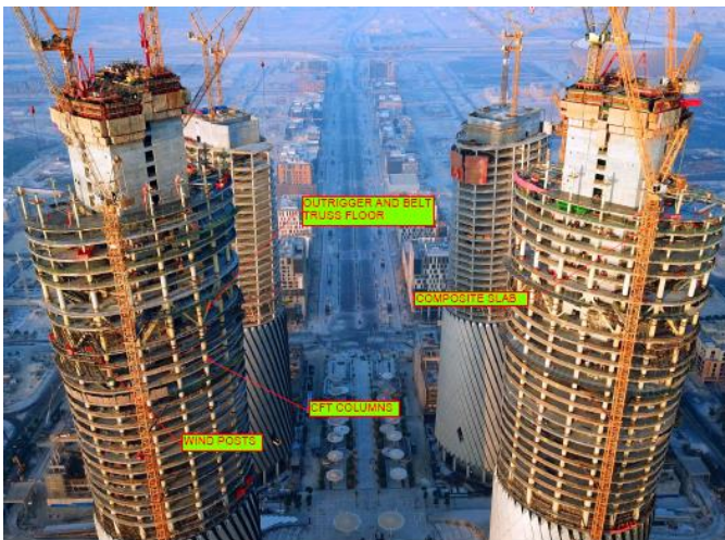
CONSTRUCTION STAGE PHOTOS (KEY ITEMS)
