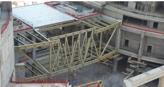
STEEL STRUCTURE TRUSS
