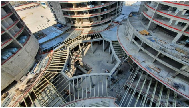
SKYLIGHT SUPPORT & PODIUM
